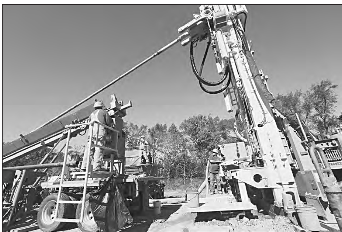
A DRILLING TEAM for the U.S. Geological Survey adds 40 feet of drilling rod to a rig as they drill down to bedrock to install a land subsidence-measuring instrument called an extensometer in northern Suffolk, Va.
