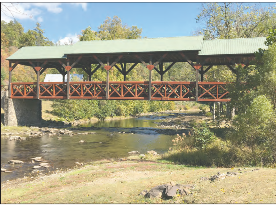
THIS BRIDGE caught the eye of Nanette Baggarly.
