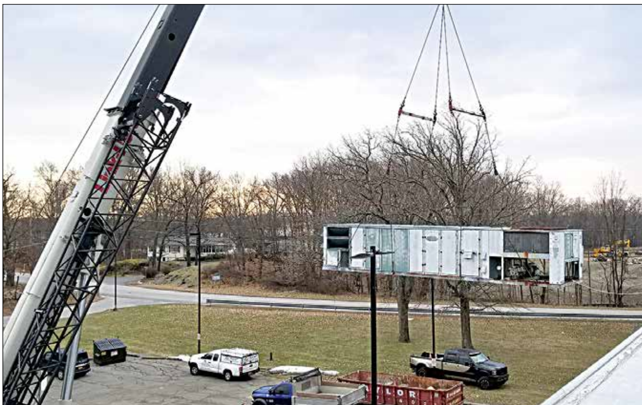
Building 112 at Montgomery town hall was stripped of its defunct HVAC system on Dec. 12, allowing the building to receive a new roof.
