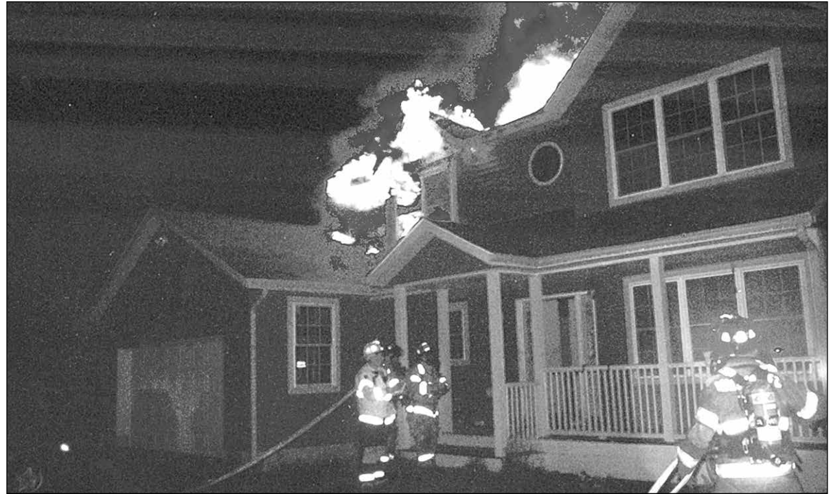
May 10, 2004: A lightning strike is believed to be the cause of a fire, Monday at 3 Knolls Road in Wallkill. No one was home at the time. Damage was reportedly extensive. The Wallkill Fire Department was assisted by companies from Modena, Shawangunk Valley, Gardiner, Walden, Montgomery and Plattekill. Several firefighters were treated for injuries. Photo by Steve Lenz.
