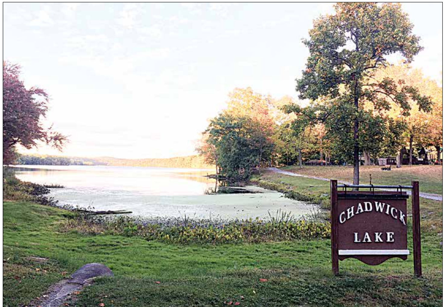
The Chadwick Lake Filter Plant will get an upgrade in 2019. The work will be carried out in preparation for the temporary shutdown of the Delaware Aqueduct in 2022.
