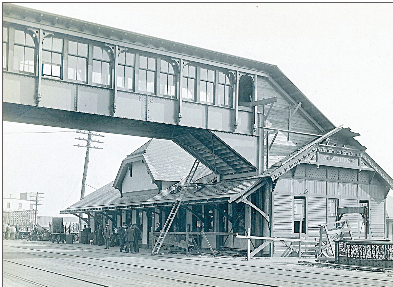
Communities started building safe overpasses like this one between Newburgh’s Union and West Shore stations.
