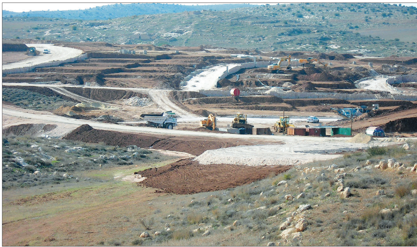
The Neta-Mirhsam site under construction.
