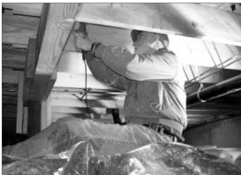
Habitat volunteer Bob Delaney installs tubing into joist pockets for the water heater.
