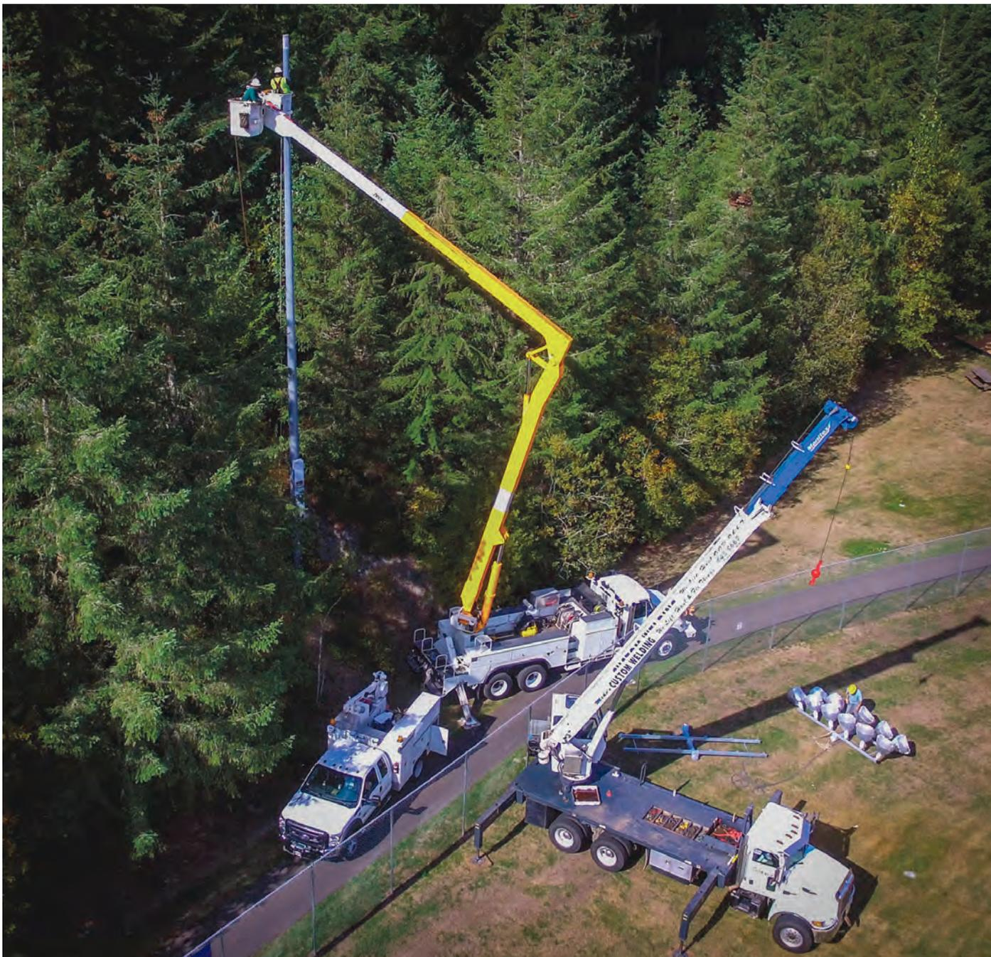
Key Pen Parks replaced the ball field lights at Volunteer Park with new LED fixtures with the help of Penlight linemen and bucket trucks to remove the old fixtures and replace them with new, brighter and more energy-efficient ones. *Photo: Peninsula Light Company*
