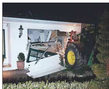
Nord-West-Media TV / Courtesy Photo A tractor stands in front of a damaged house after it broke through the wall in Buende, north-western Germany today. Unknown intruders steered the tractor into the house and broke through the wall in order to steal a safe. The residents were not injured.
