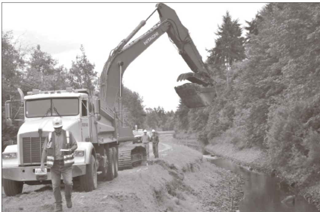
Employees of Dulin Construction, Centralia, work this week to repair a sinkhole in a canal near Yelm that powers Centralia City Light's hydroelectric plant on the Nisqually River.
