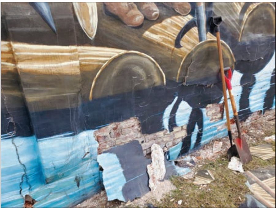
The mural has outlived its lifespan and parts of it are cracking, chipping and crumbling off.
