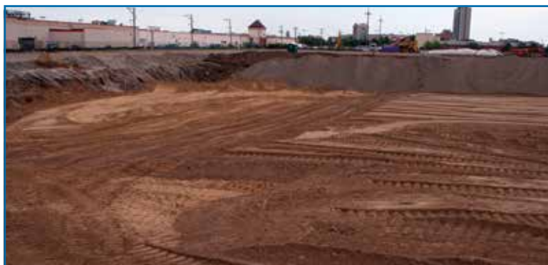
Work at the soccer stadium site is well underway. The $10 million building permit issued July 14 is for excavation, site work and footings only.
