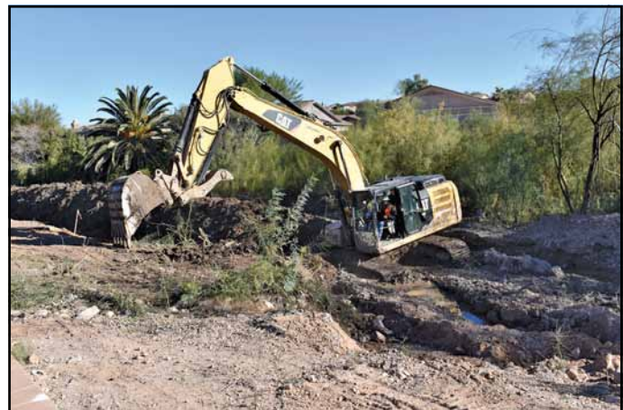
A large shovel works along the drainage channel in Panorama Wash on a drainage improvement project.
