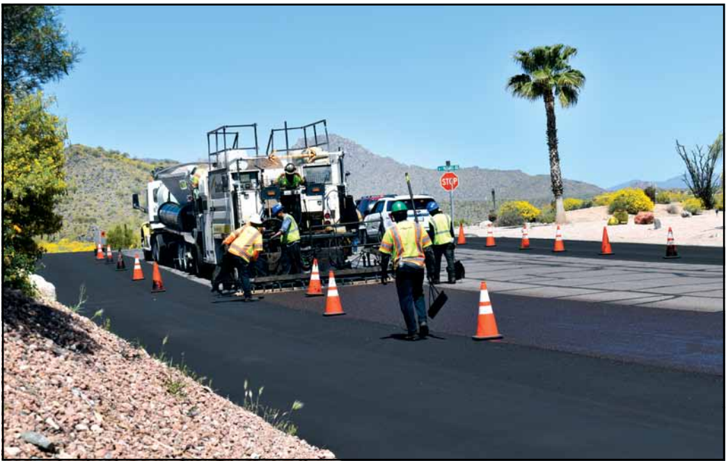
Slurry seal, like this recently laid over the asphalt on El Lago Boulevard, is part of the process to keep streets well maintained.
