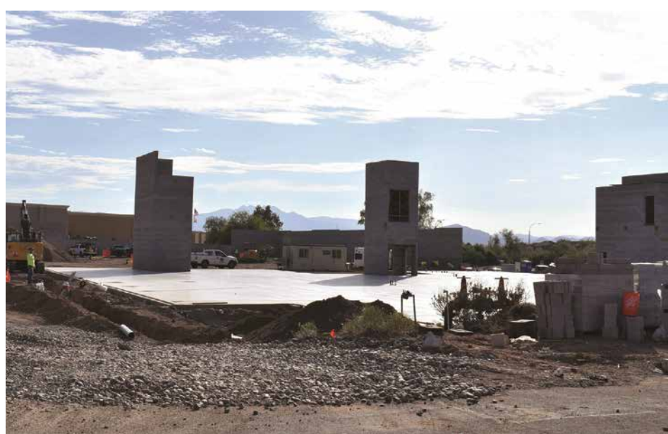
STORAGE BUILD GOING VERTICAL
