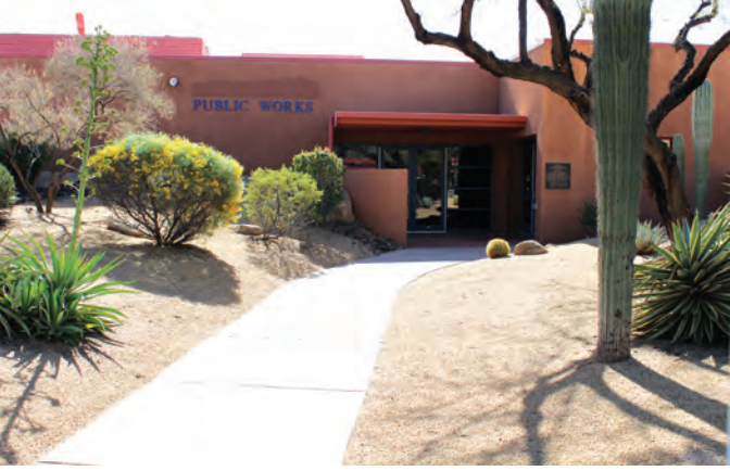
The Town of Paradise Valley Public Works building is across the parking lot from Town Hall.
