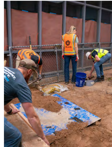
Workers from Okland Construction and Banner Health help renovated a pond on the Cactus High School campus in Glendale March 28. (Courtesy Erin Dunsey/Peoria Unified School District)
