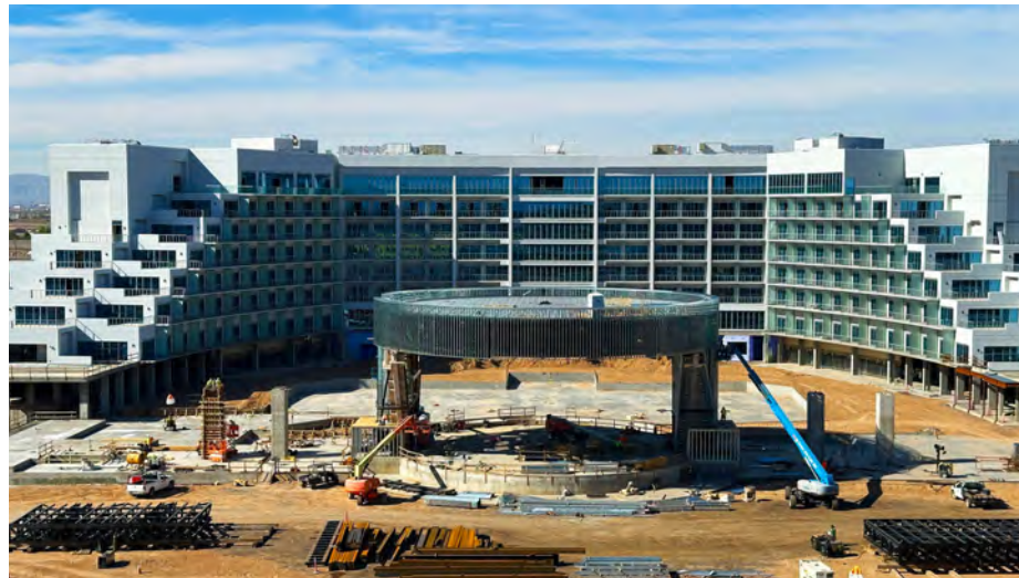
Construction crews work on the VAI Resort in south of State Farm Stadium in Glendale in November 2024. Two Glendale City Council actions related to the project were sent to Glendale voters to decide on in a special election May 20. Voters rejected Proposition 401 and approved Proposition 402. (Courtesy VAI Resort)
