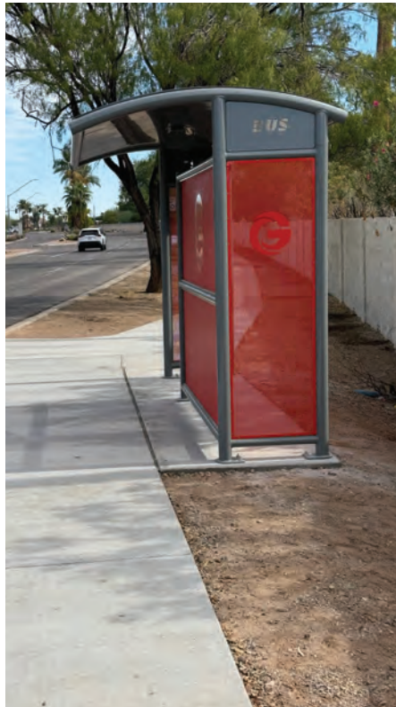
This shaded bus stop seating area on eastbound Union Hills Drive near 67th Avenue has been built from scratch in the past year by the city of Glendale. (City of Glendale)
