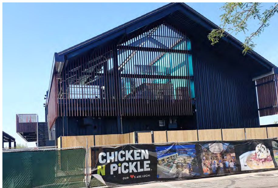
The Chicken N Pickle location at Westgate in Glendale is seen under construction in the summer of 2023. (Independent Newsmedia/Steve Stockmar)
