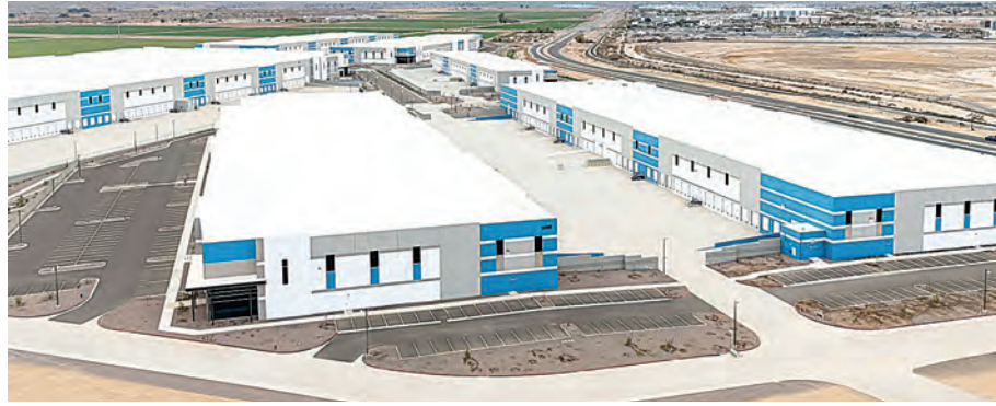
Lincoln completes first phase of Goodyear AirPark and begins its development on a retail expansion. (Submitted photo/Stacey Hershauer)
