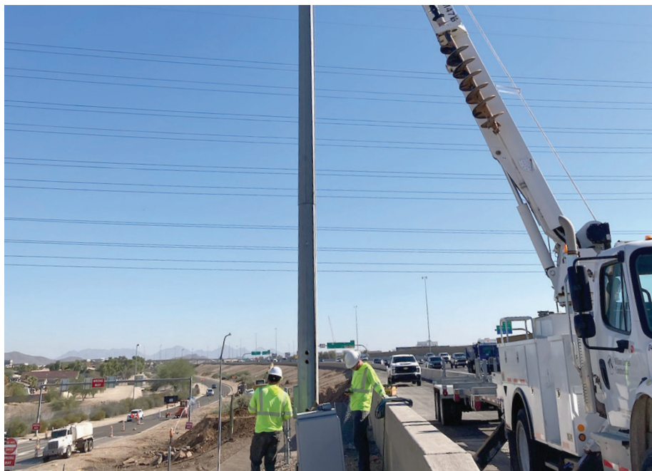
Construction workers install an element of the Loop 101 expansion, a $140 million Arizona Department of Transportation project. (Courtesy ADOT)
