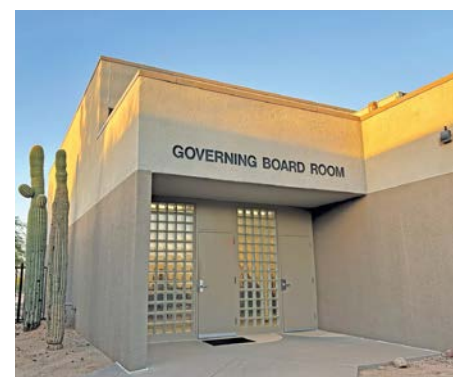
Cave Creek Unified School District's governing board building 33016 N. 60th Street, Scottsdale. (Maya McFall/Independent Newsmedia)
