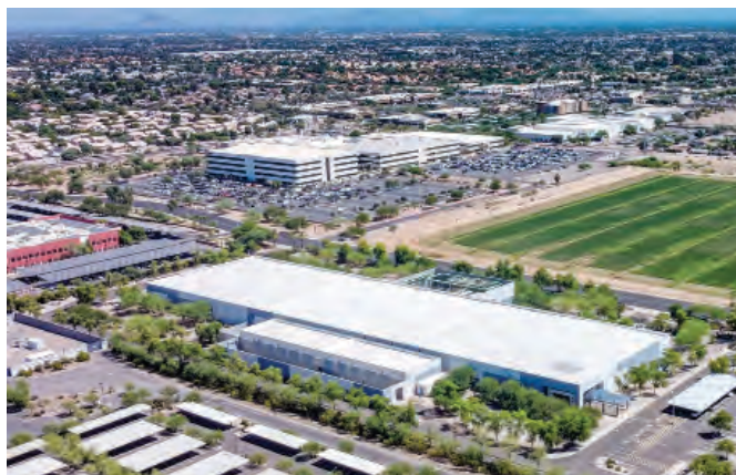
Commercial real estate firm Lincoln Property Co. has announced the purchase of a 191,000-square-foot, partially occupied data center on 14.5 acres at 2500 W. Frye Road in west Chandler. (Courtesy of FocusAZ)
