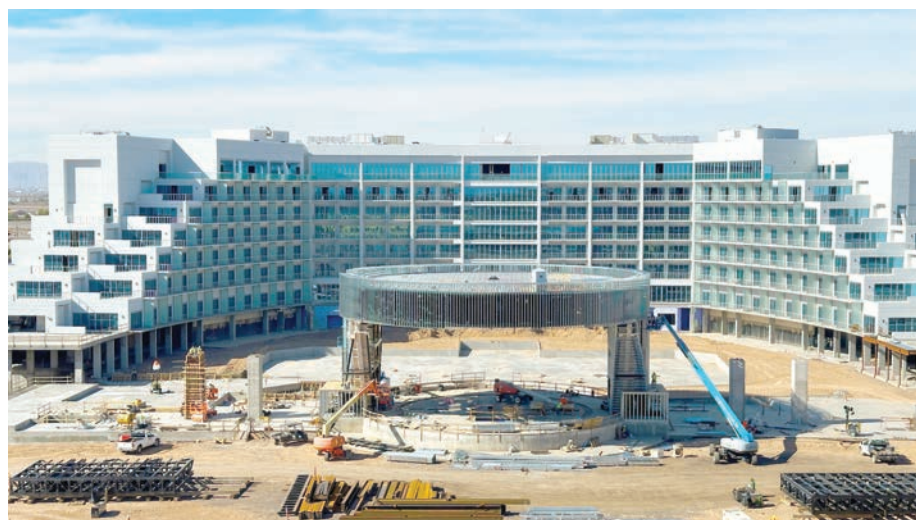
Construction crews work on the VAI Resort south of State Farm Stadium in Glendale this past November. Both the resort and the Mattel Adventure Park included in it have been delayed to a 2026 opening date after plans to open in 2024 and 2025. (Courtesy VAI Resort)
