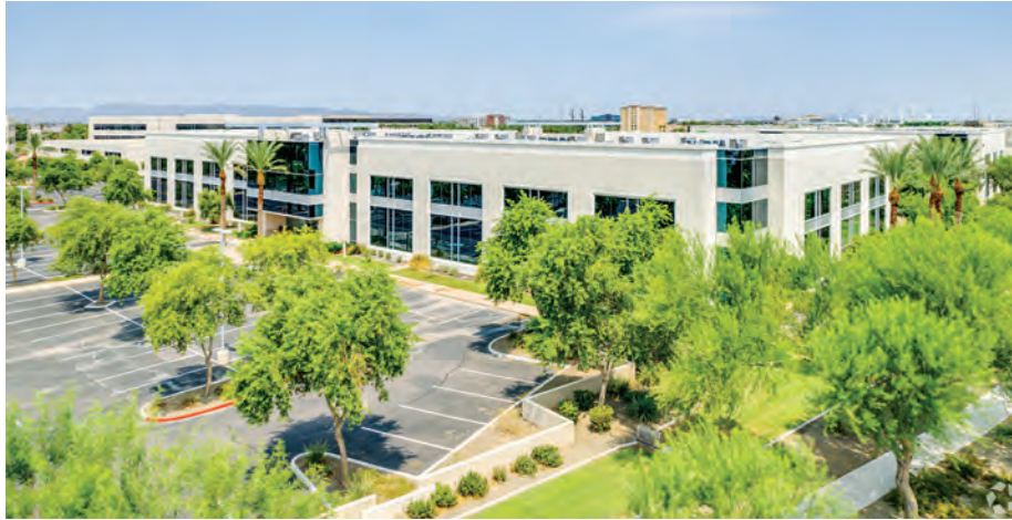
Rosendin, a national employee-owned electrical contractor, has announced the purchase of Allred Park Place Building 4 in Chandler, in a business park near Spectrum Boulevard and Willis Road, in the Price technology corridor. (Courtesy of Rosendin Electric, Inc.)
