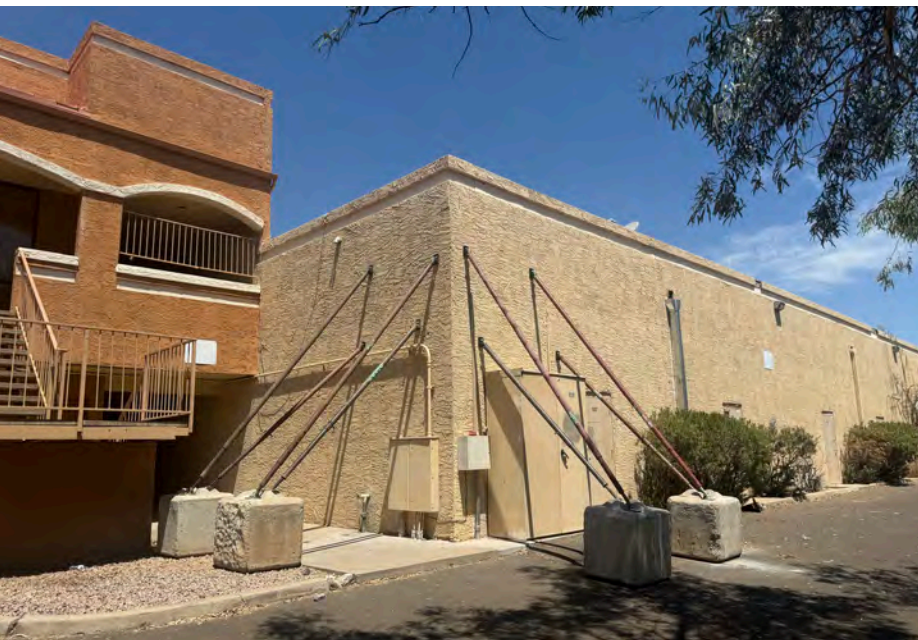
Temporary structural supports in the back of Del Prado Plaza allowed tenants to move back in. (Independent Newsmedia/Tom Blodgett)
