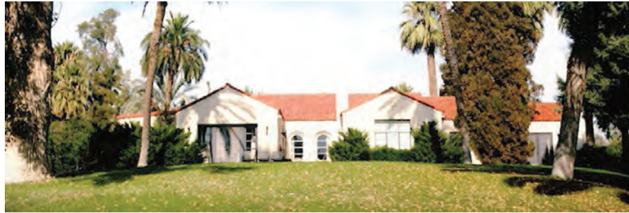
Exterior face-lift moves forward as founder's homestead awaits federal historic district designation. (Submitted photo/P.W. Litchfield Heritage Center)
