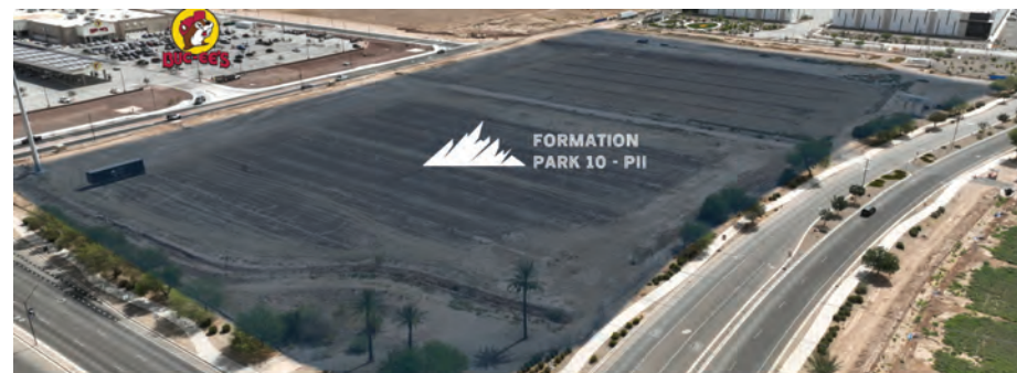
A new buildout along Interstate 10 will add three new buildings, completing a 44-acre business park. (Submitted photo/Formation Interests)
