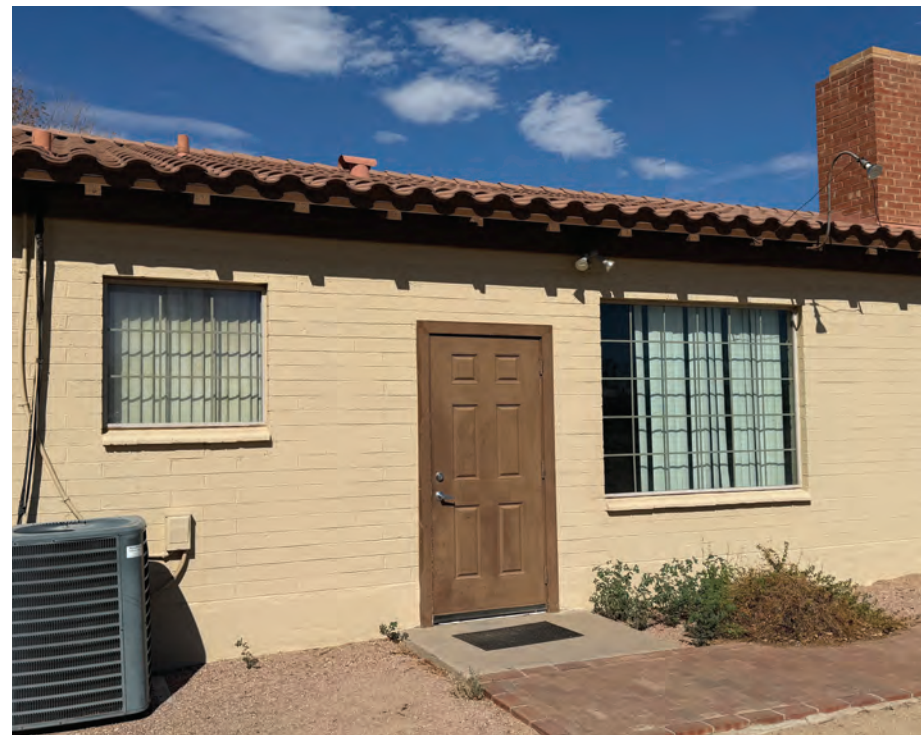
The current Litchfield Park Scout Lodge at 299 W. Fairway Drive. The city has identified the property as the site of a possible future parking garage, although demolition has not been formally approved. (Noah Flug/Independent Newsmedia)
