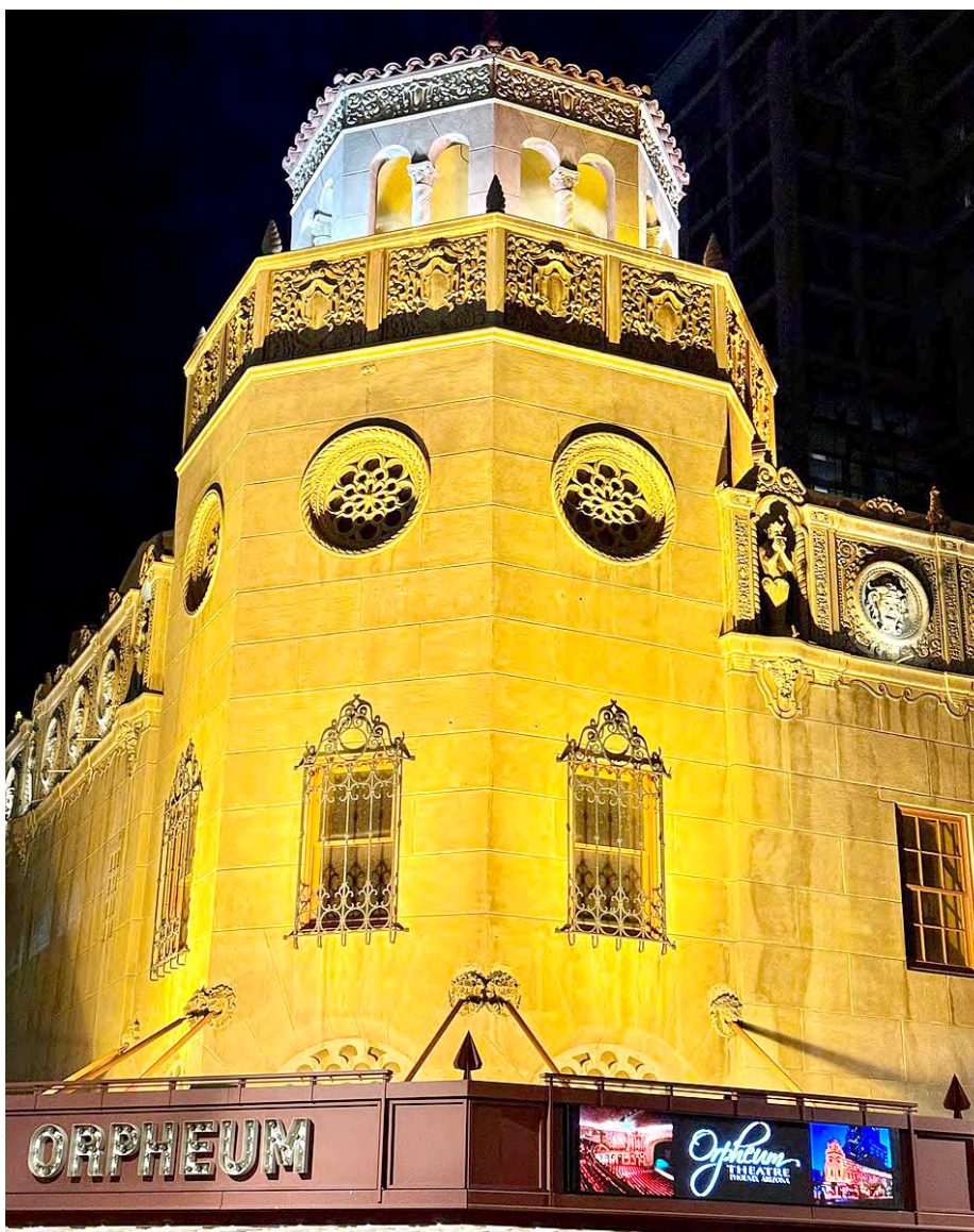
The historic Orpheum Theatre's past will be told through guided tours Oct. 23-31 to highlight its architecture, backstage spaces and reported ghostly encounters. (Photo by w_lemay, provided by Wiki Commons)
