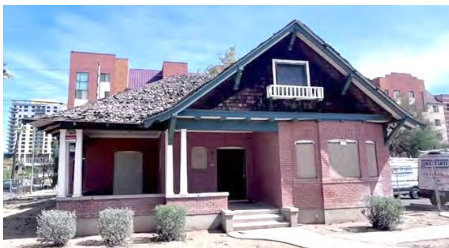
The 117-year-old Sargeant-Oldaker House in Phoenix is being relocated just a few dozen feet to the corner of the property it sits on so that the property owner can build multifamily housing on the rest of the property. (Submitted by the City of Phoenix)
