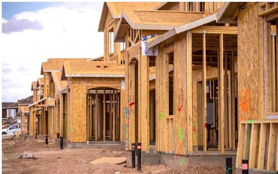
Homes under construction in Queen Creek can now continue as a state judge ruled the Arizona Department of Water Resources improperly changed a rule regarding the need for a 100-year water supply for new development. (Special to Independent Newsmedia/Arianna Grainey)
