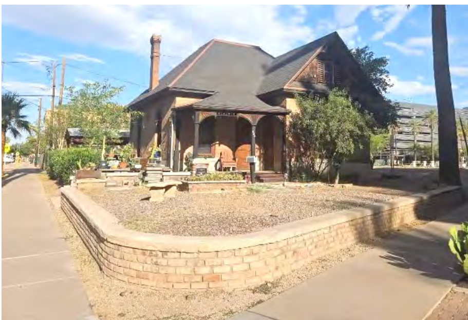
The 124-year-old Louis Emerson House, at 623 N. Fourth St. in downtown Phoenix. (Submitted by the City of Phoenix)
